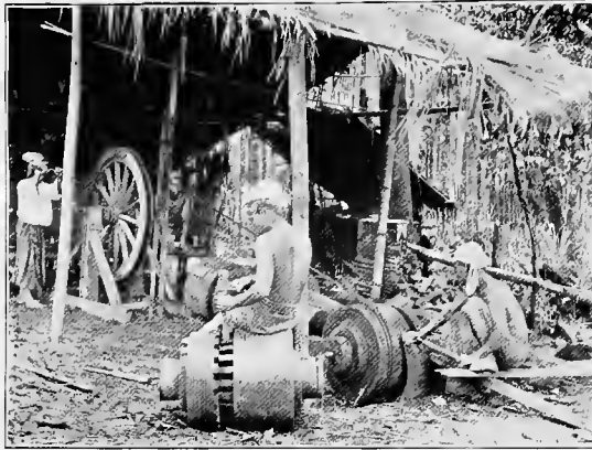
187. TURNING ROLLERS FOR THE CANE-MILL.
